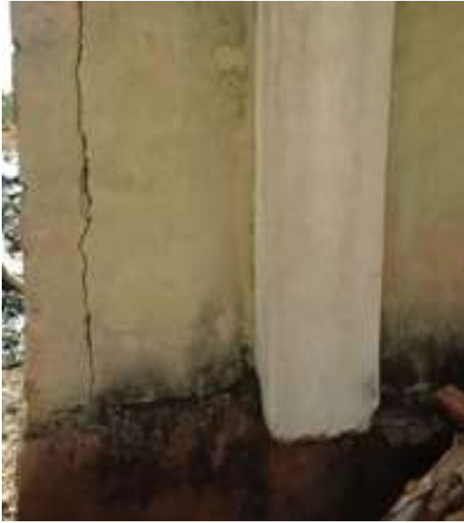
Figure 3: Vertical cracks
